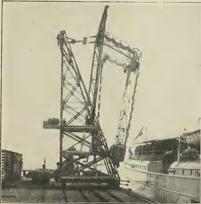
more than 2 horsepower for its operation while at normal speed carrying forty-two bunches of bananas per minute. With the use of this machine the delay and drudgery by human labor are reduced, as well as the cost of loading and unloading cargoes. Vessels are now got out of the way in less than half the time than when the bananas were handled entirely by human efforts and passed into and out of the ship's hold from man to man.
